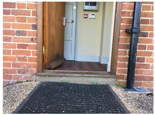
To get into the cottage there is a step up off 100mm by depth of 170mm with a step down of 60mm
