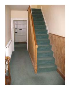
Stairs to first floor -13 risers at 190mm. There is a banister/handrail to one side at 900mm and carpeted stairs. This area is well lit.
