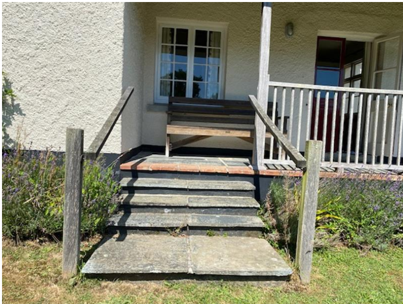
Entrance onto veranda to sitting room
