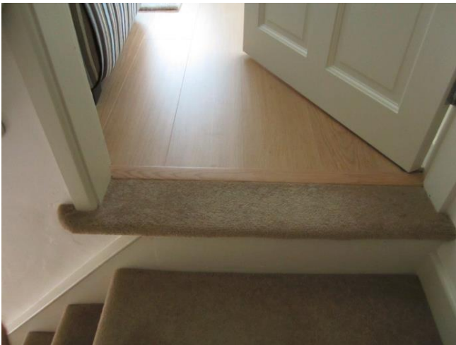
Step at top of stairs into lounge
