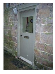
• Back door opens to 800mm wide and with a 20mm threshold
