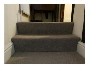
• Bedroom door 800mm wide with an uneven threshold of 40mm
