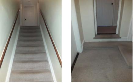
Approached from entrance lobby directly to carpeted staircase with handrails either side -13 steps of 210mm depth x 190mm height x 860mm width.
