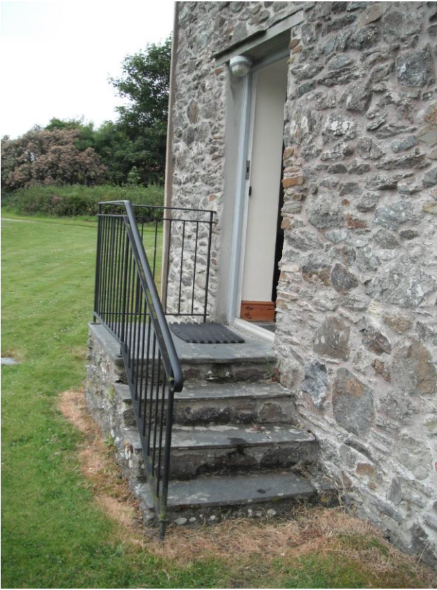
Door from back hall leading to garden
