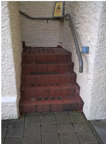
External steps up to the apartment.
