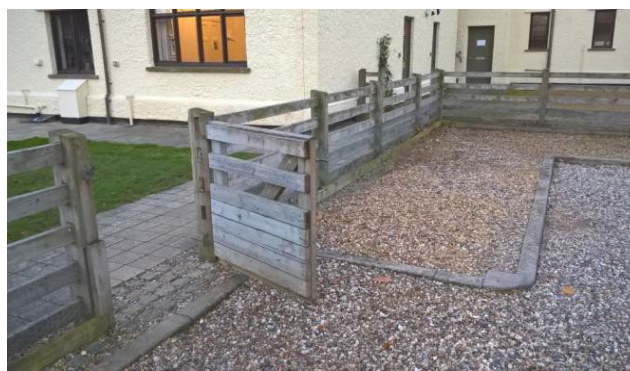
Gate from parking area to path base of steps
