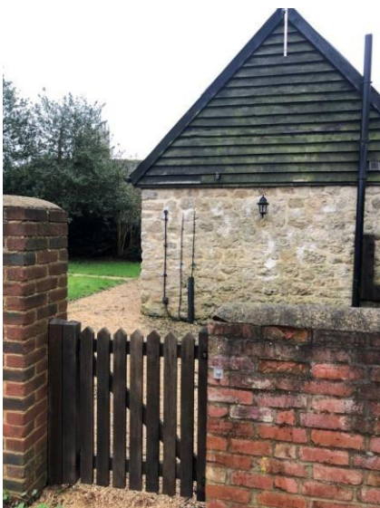
Path from parking to cottage entrance
