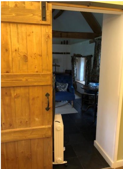
Main room/ bathroom doorway
