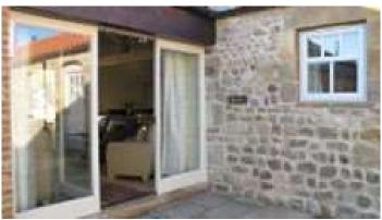
Entrance in shared courtyard, Step up to threshold 150mm with a 30mm weather bar, door is 900mm wide
