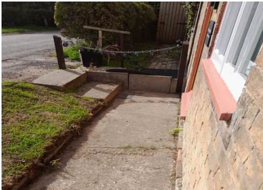
Level path to front door/steps down from Lode Lane
