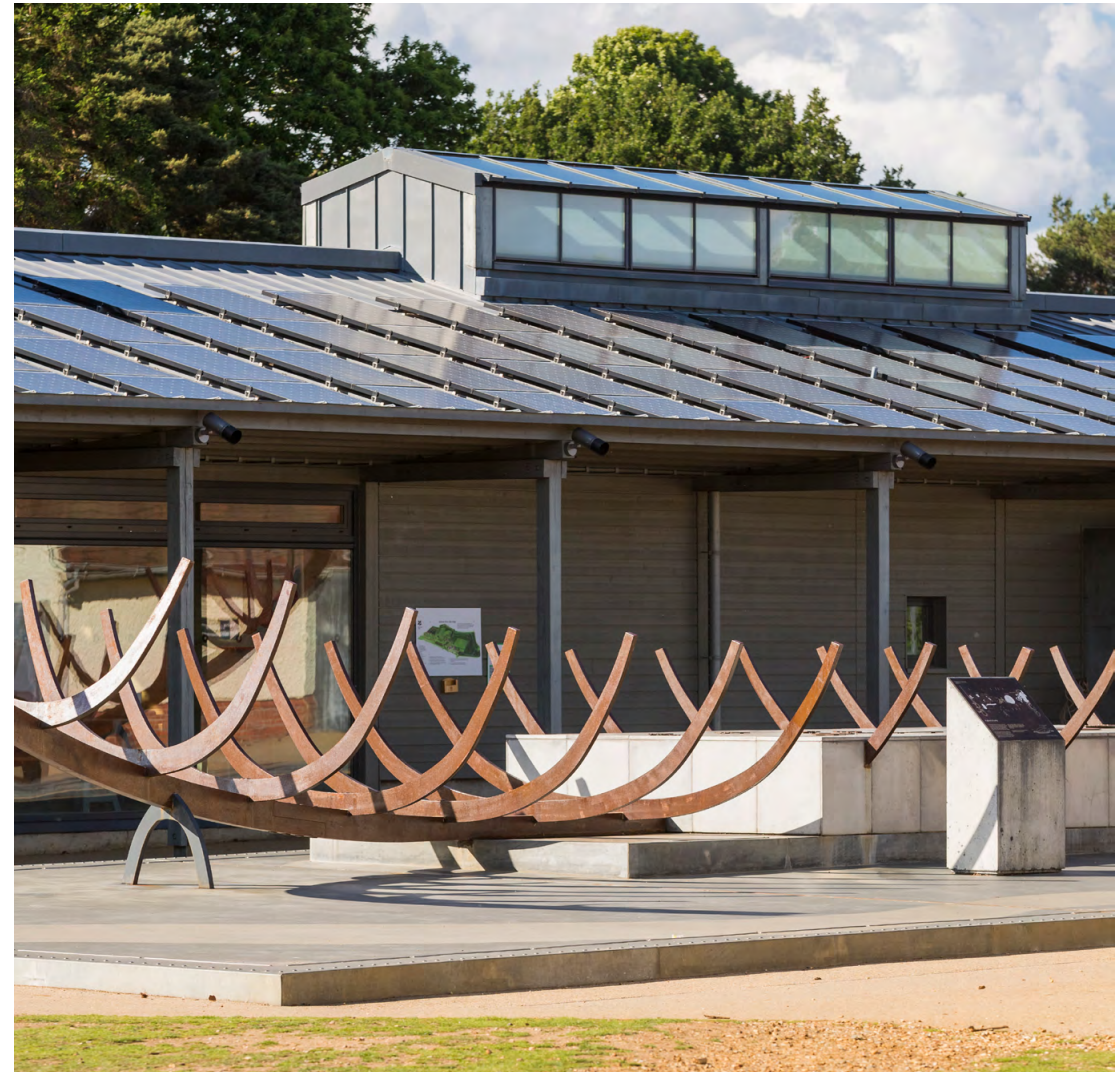
Photovoltaic panels at the visitor centre, Sutton Hoo, Suffolk.
