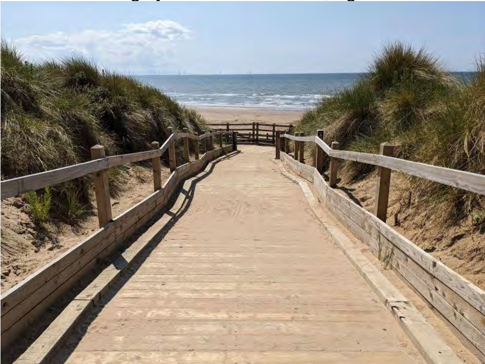
Revetment and handrail on wooden boardwalk, looking west
