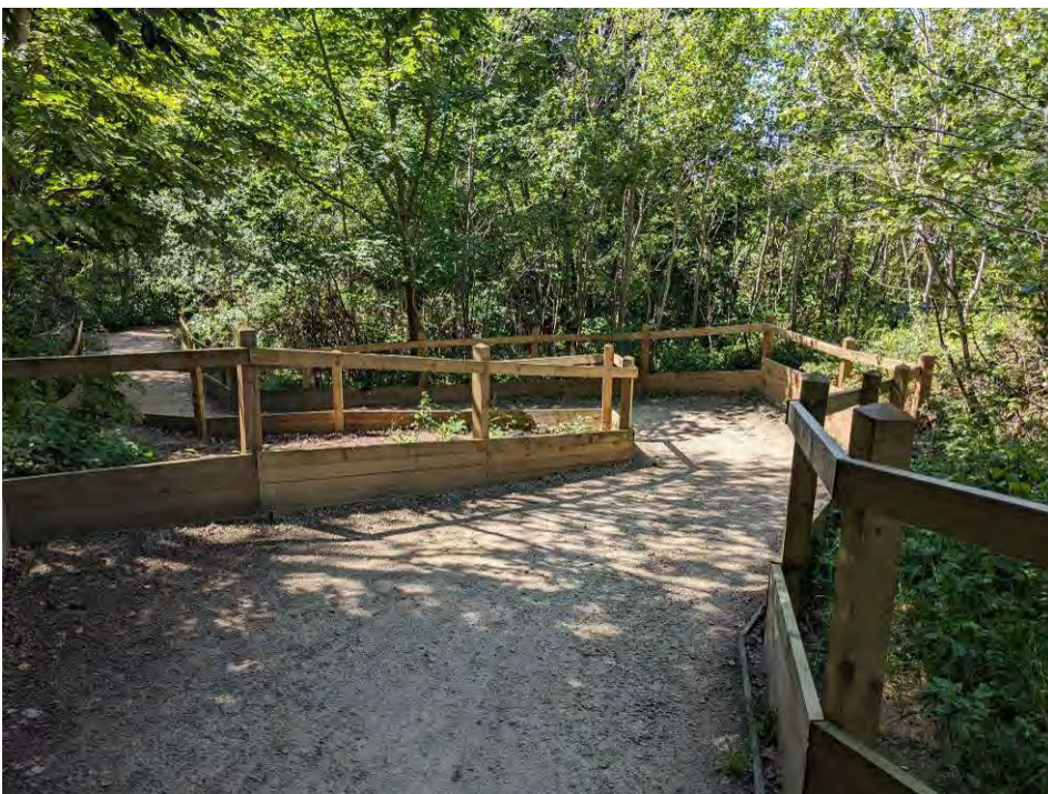
Path and revetment with handrail on Kirklake Path, looking west
