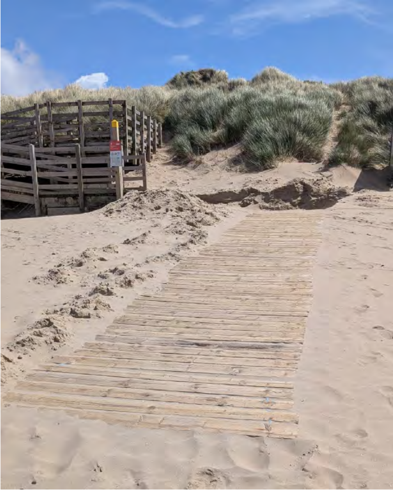
Wind-blown sand on the roll-out boardwalk planks on the beach, looking east
