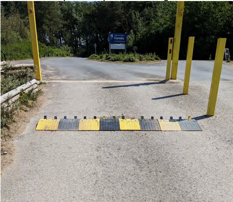
Flow plates at Lifeboat Road car park as you leave site, looking south
