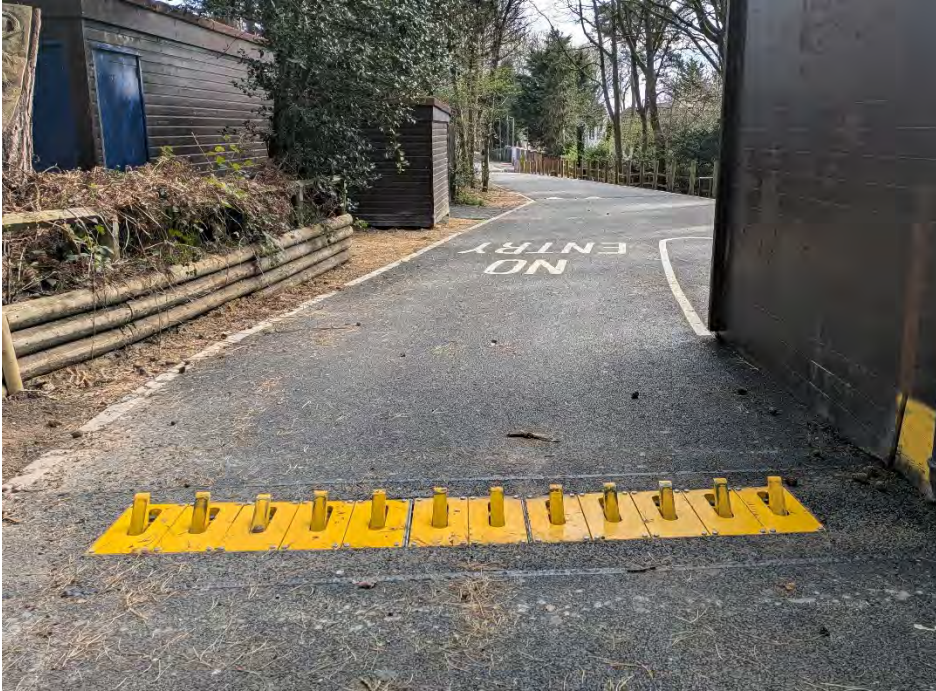
Flow plates at Victoria Road car park as you leave site, looking east
