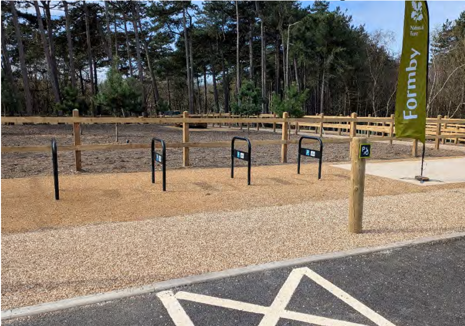
Cycle racks at Victoria Road car park
