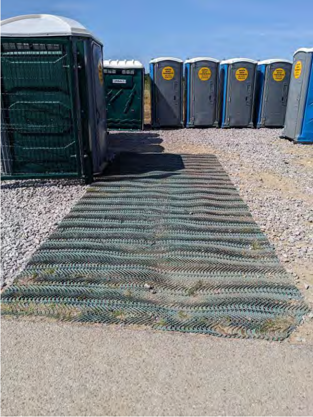
Plastic mesh that connects the tarmac to the portable toilet with accessible features
