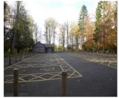
Accessible parking area
