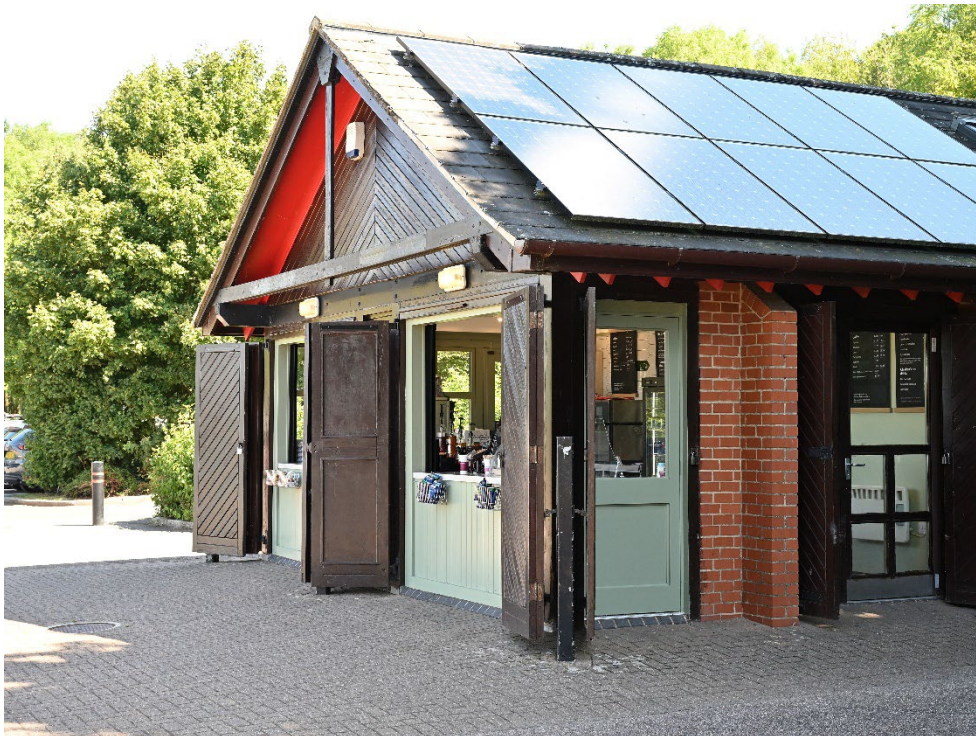
Photo 5 Refreshment kiosk near the main car park
