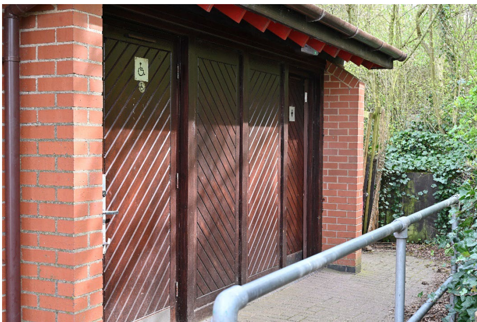
Photo 3 Entrance to accessible toilet
