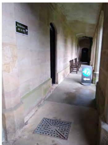
Entrance to the changing place
