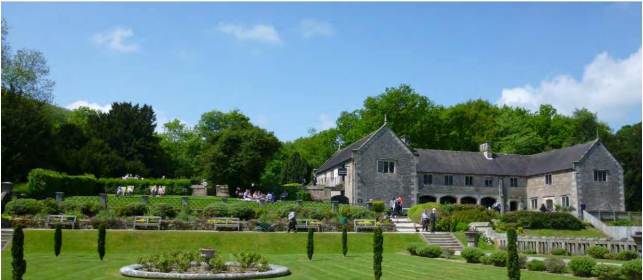
View of the Italian Garden, with the stable yard facilities on the right
