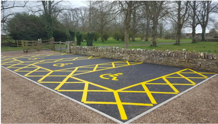
Image 1: Designated disabled parking space.
