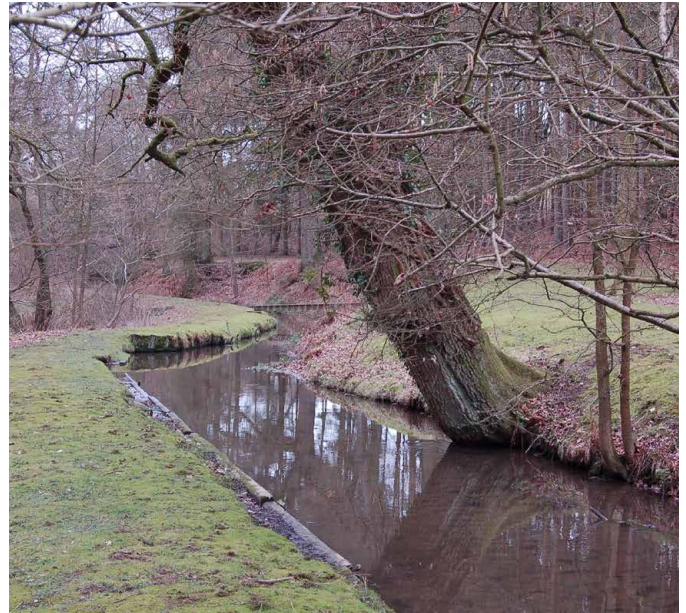
^ This example at Chilworth in Surrey shows the erosion on the outer curve of the canal and the potential damage from a collapsing tree
