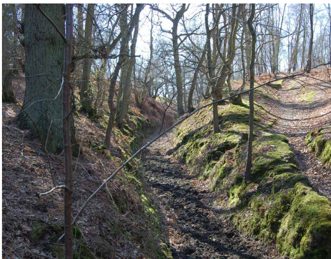
^ Only a winter photograph can show the extent of erosion of this common boundary bank and the lesser damage to the higher level path
