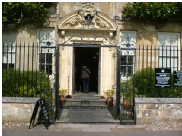
Main entrance door in to Visitor Reception
