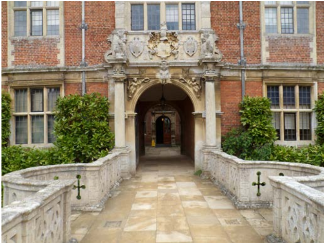
Old Moat bridge showing hall front door
