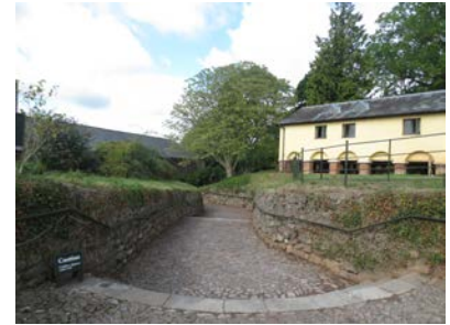
Cobbled path with handrails and steps down to Visitor Reception
