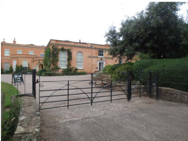
Metal gates at end of the path to access house
