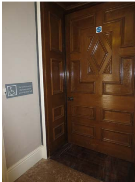
Large wooden door with sign for bell on left if required
