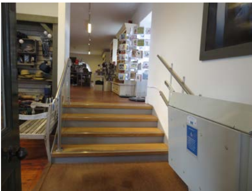
Steps and wheelchair lift to main sales area in shop
