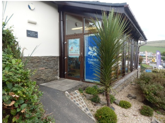
Rear entrance - level access
