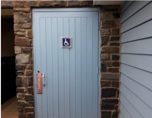
Entrance to accessible toilet
