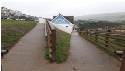
Access ramp to toilets
