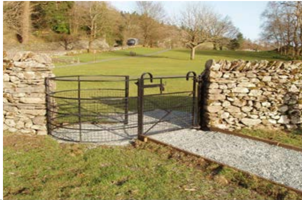
Access gate with RADAR key from Borrans Park.
