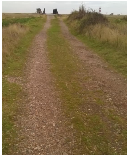
The track leading to the Bailey Bridge
