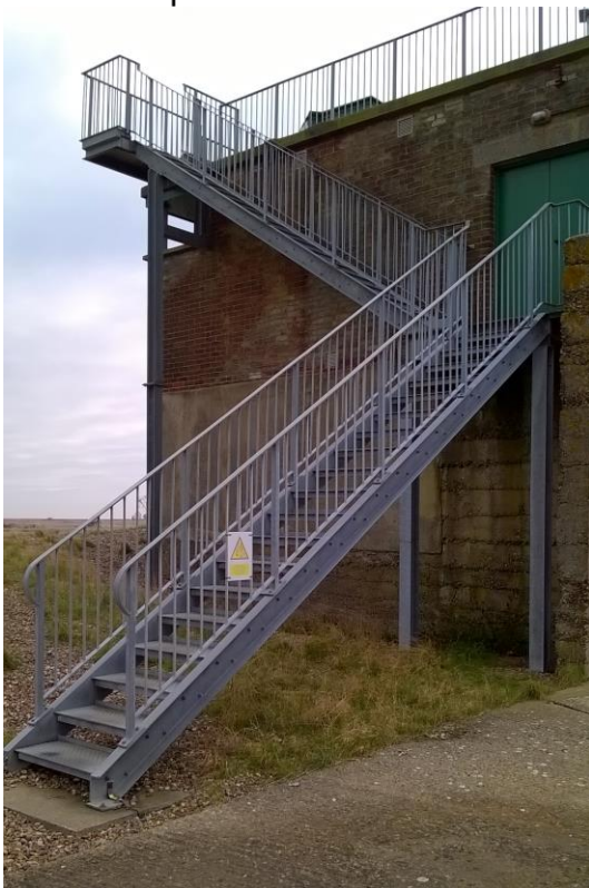
Steps to the main floor and roof of the Bomb Ballistics building
