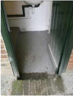
Entrance to outside toilet
