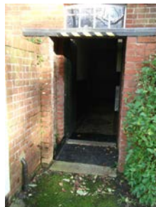
Side entrance door
