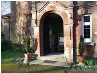
Front entrance door
