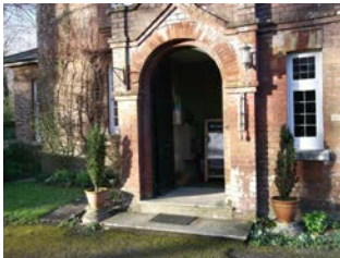
Front entrance door
