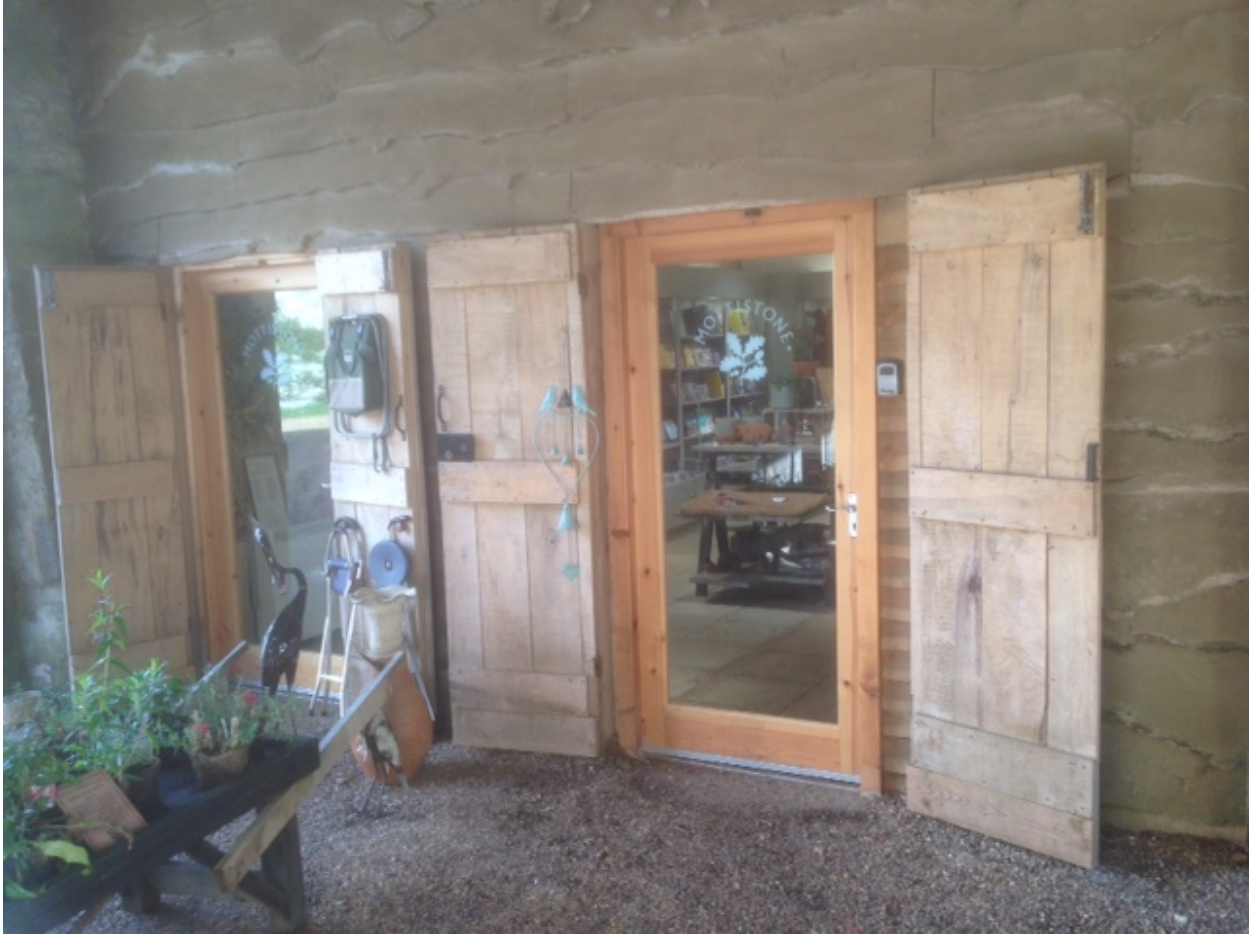
Visitor Reception Entrance ( Right hand door ) Exit ( Left hand door )
