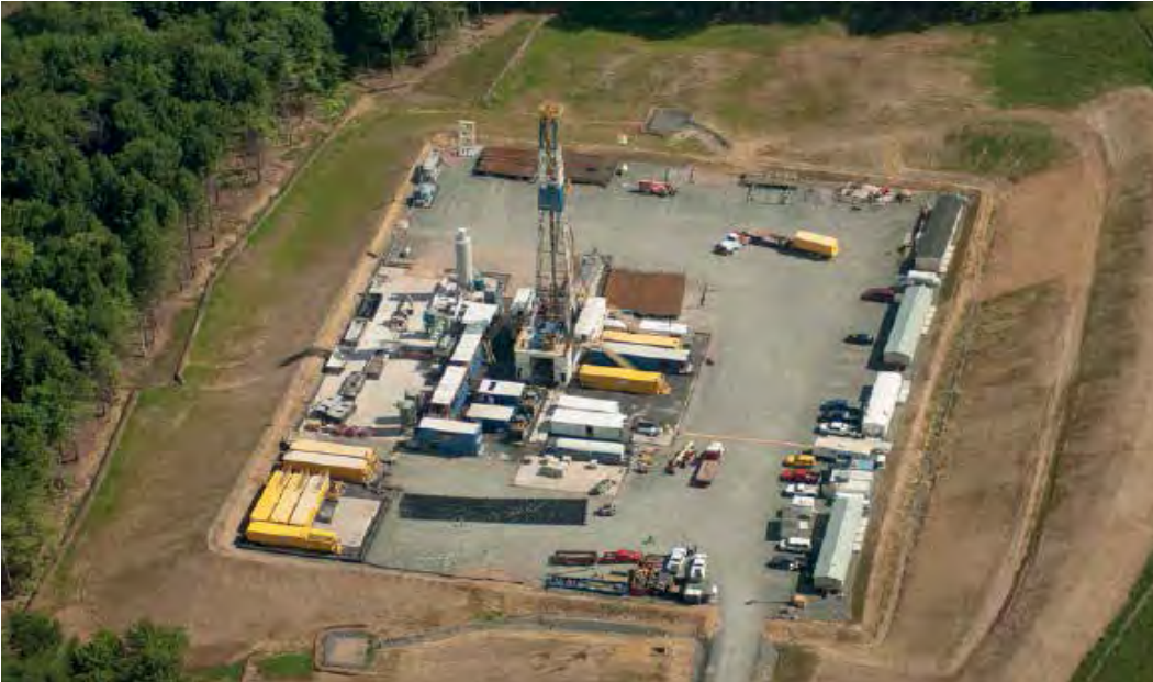
Methane leakage should be monitored across the whole site
