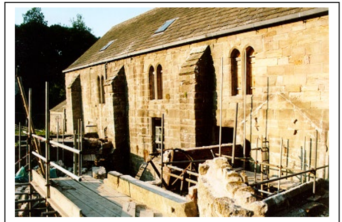
The Mill during restoration work.
