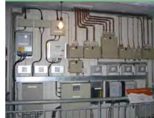
Energy control board for integrating hydro-generated electricity, solar-generated electricity and battery storage. The control panel also allows visitors to monitor the site's power generation and usage
