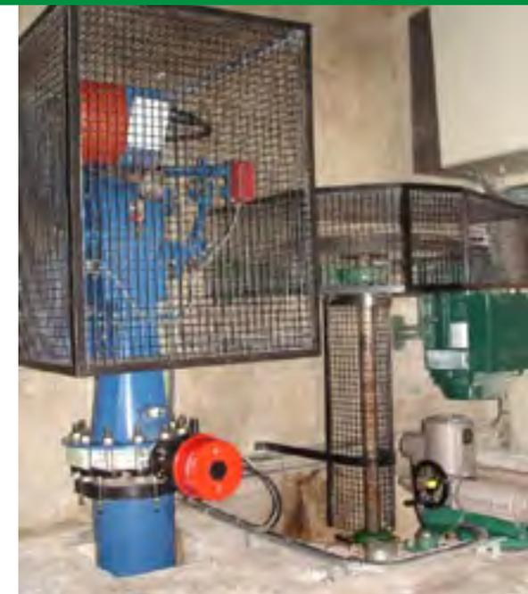
The refurbished 1926 hydroelectric turbine and the new 1.5kW turbine for low water levels
