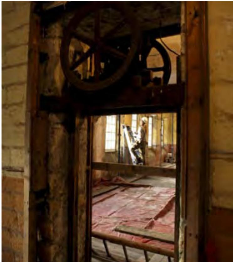
The interior during restoration works. The mechanism of the dumb waiter is in the foreground.
