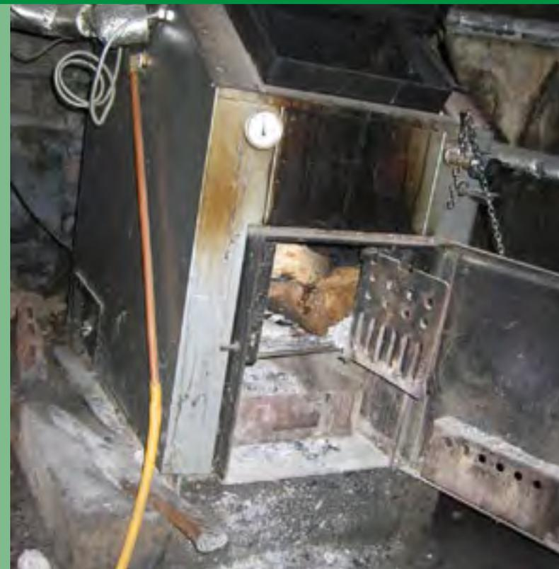
The 60kW downdraught log-burning boiler installed in the former engine house, supplies hot water to the café
