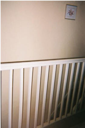
Rail between bedroom and stairs
