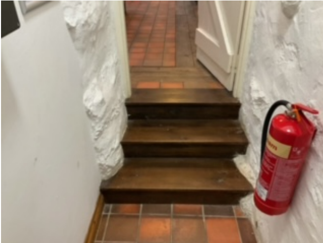
Lower ground floor access.
