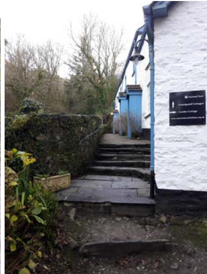
Steps from car park area
