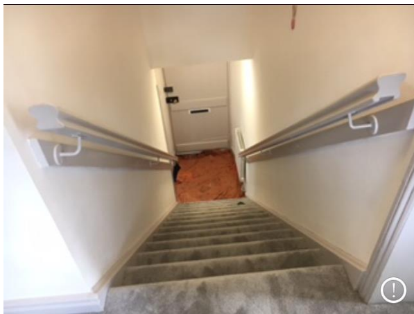
Staircase and handrails (protective cover at door)
