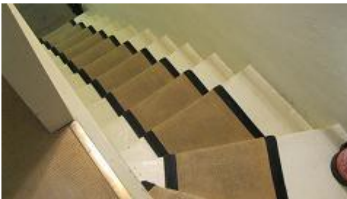
View of Staircase to first floor from top and bottom
