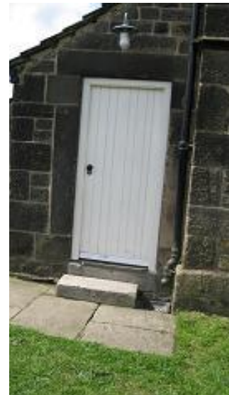
Entry door into cottage
