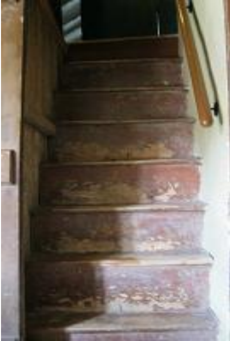
View From Bottom of Staircase
