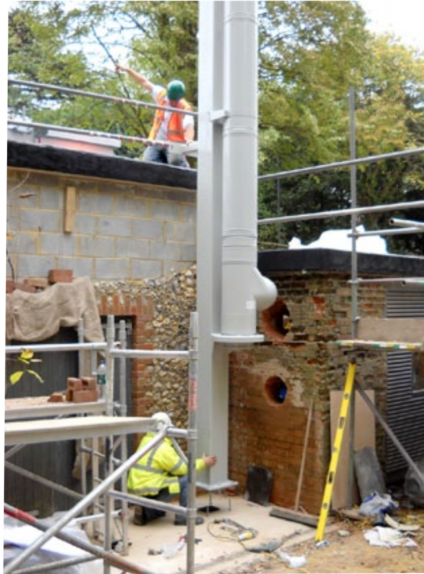
Above Flue being lowered into position
