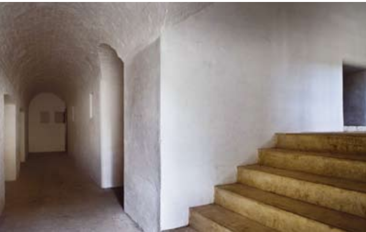
Inside the Magazine at Reigate Fort
